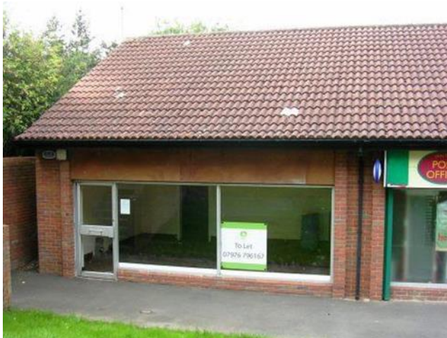
Figure #1 – premises store front
